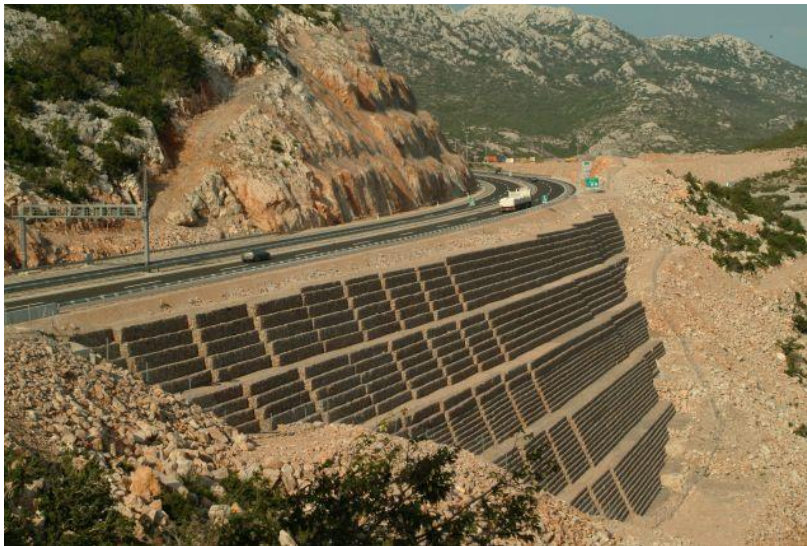
Figure 1: Gabions as support for a multi-lane roadway, Sveti Rok, Croatia (from Wikipedia, https://commons.wikimedia.org/wiki/File:SvetiRok.jpg ).
