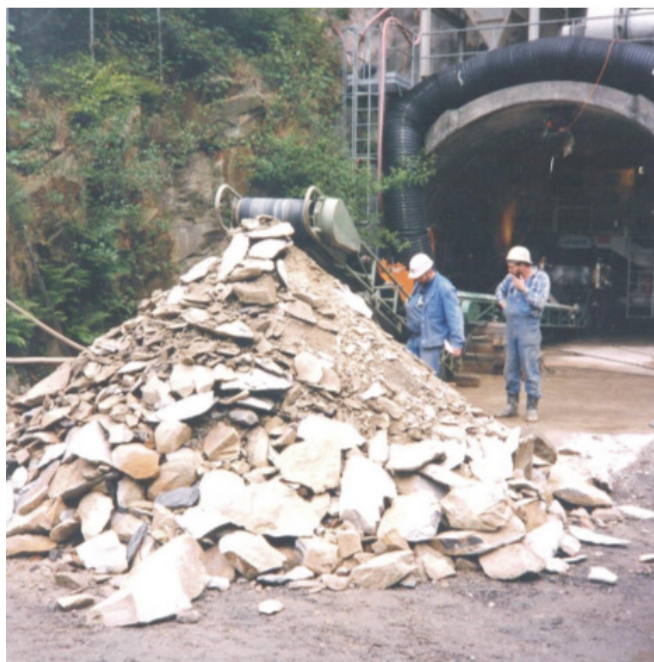
Figure 5. Rock cutting produced by CMM in Ruhr Sandstone.
