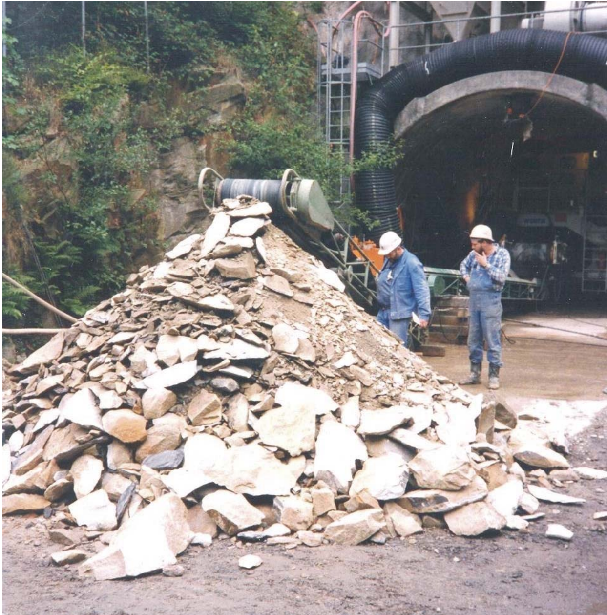
Rock cuttings produced by CMM
