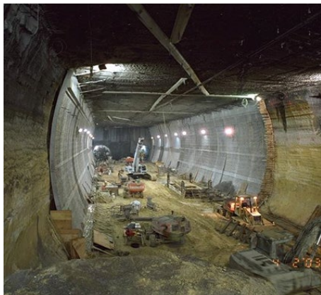
LRT station during construction.
