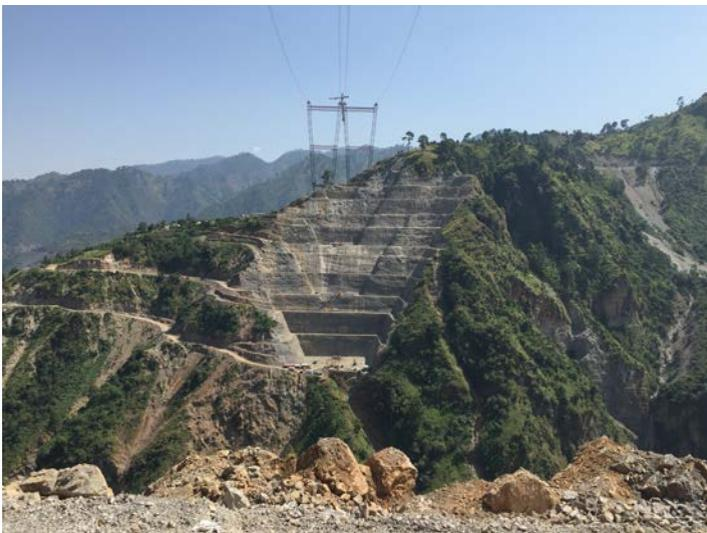
*Bakkal end of the valley, after excavation for the arch bridge abutment.*
